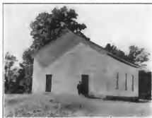
MOUNT PISGAH CHURCH, NEAR BANCROFT
